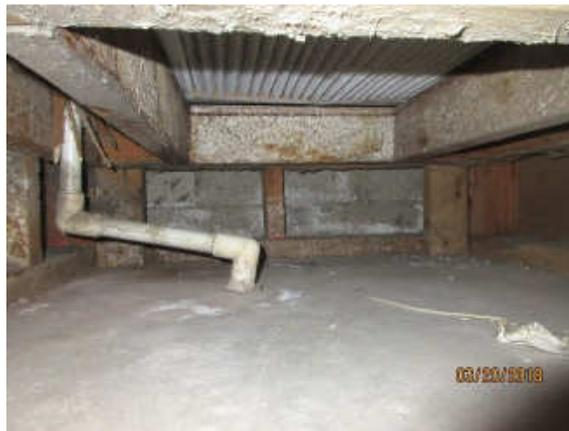
*Efflorescence on retaining wall below HVAC*
