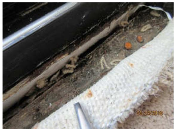
*Mold growth on tack strip and subfloor in front of slider*
